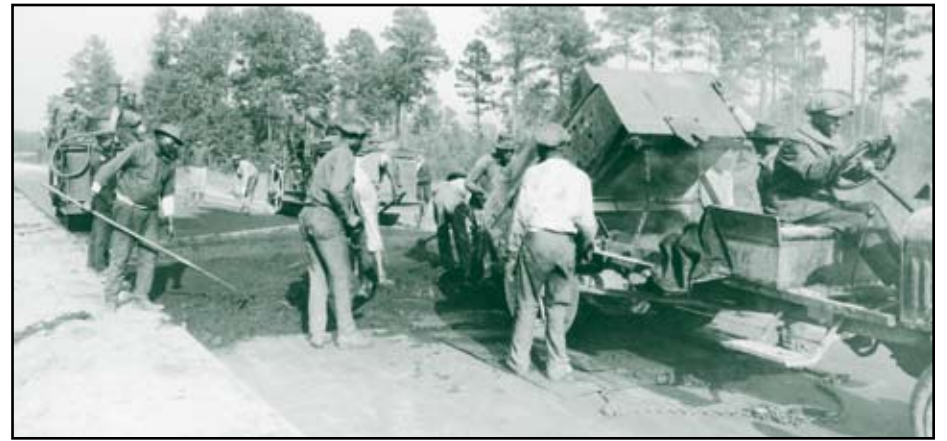
Dumping hot-mix asphalt. Photo Courtesy NAPA
